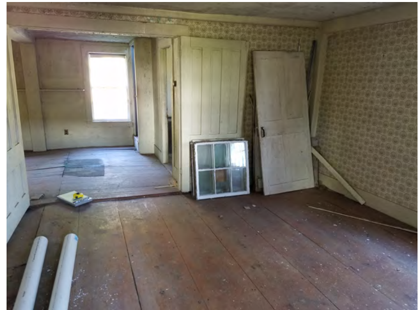
Historical sash stored in the house
